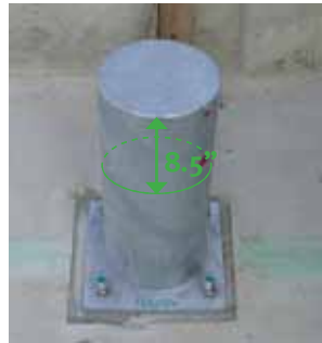
Stanchion davit pedestal base. NOTE: There must be at least 8.5 in. from top of base to finished roof to allow clearance for adapter.
