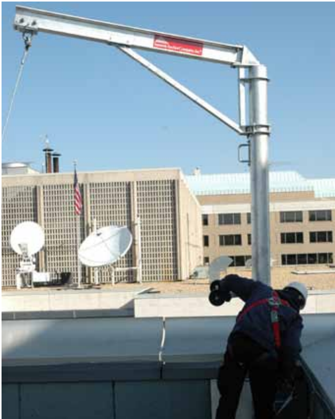
Davit Mast is locked into place once hoisted upright.
