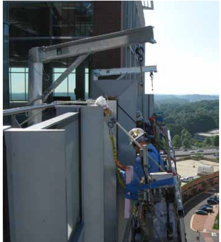
These ground-rigged, portable davits prevent loading on a glass parapet wall during suspended maintenance.
