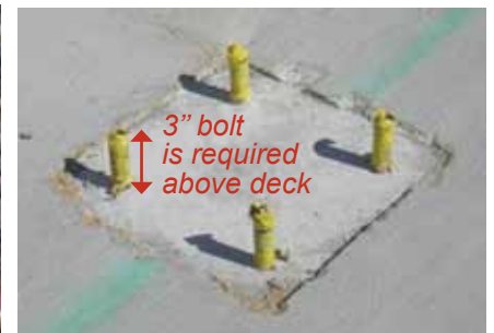
SM-DVT-CGE: Davit cage before and after pouring of concrete slab.
