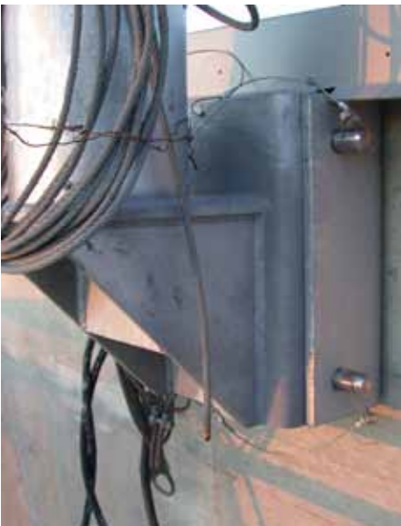
SM-DVT-SKT-W: Davit socket is attached to the wall davit pedestal base. Davit arm is inserted into the davit socket.
