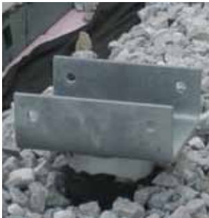
Formed Plate davit pedestal base
