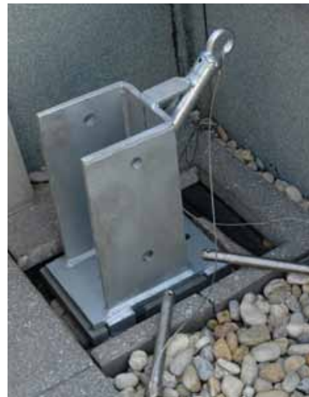
SM-DVT-SKT-R: Davit socket is attached to the recessed davit pedestal base. The davit arm is then attached to the davit socket.
